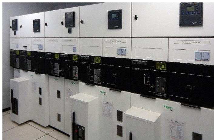
Pic. 3: Medium-voltage cells
