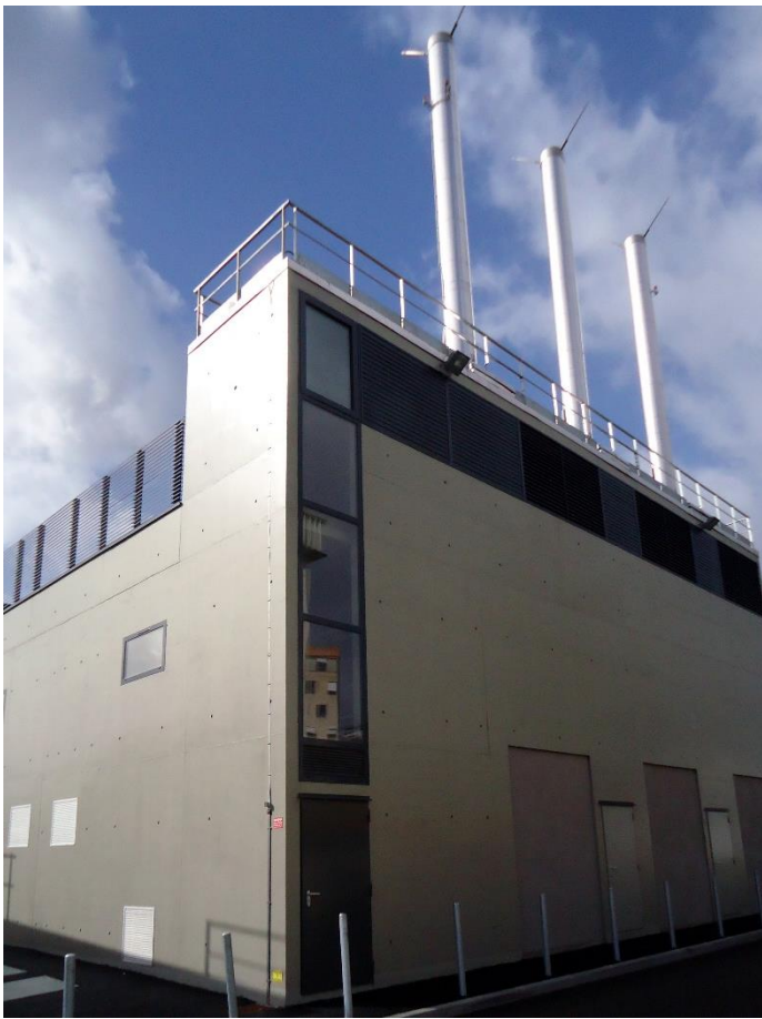
Pic. 4: Premises of 350m 2 containing the generators
